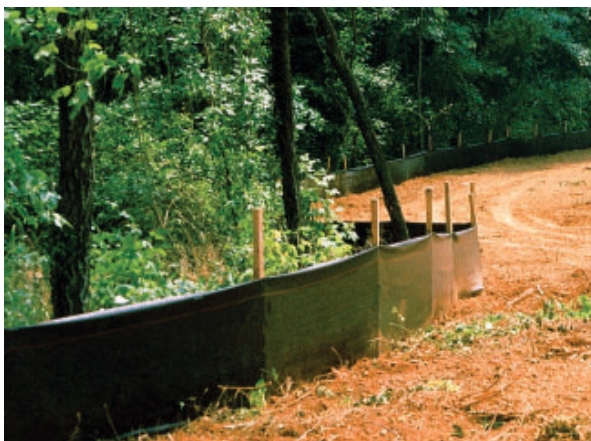
Photo 2 Example of a Silt Fence
