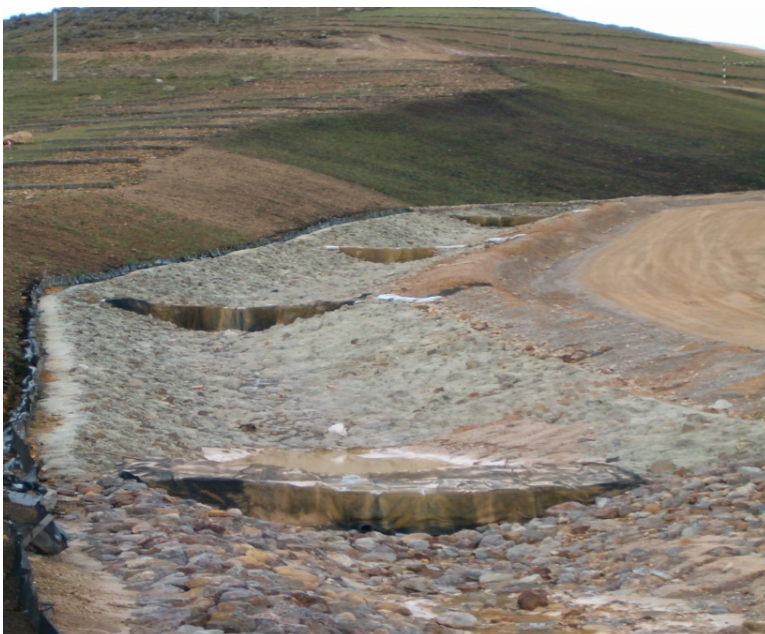
Photo 4 Example of a Check Dam
