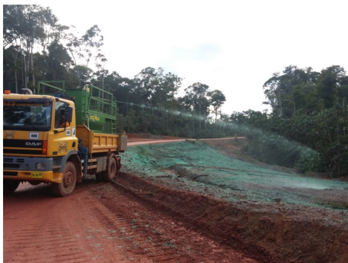
Photo 3 Example of Hydromulching
